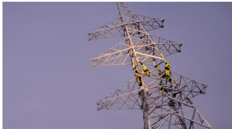
**Montaža i podizanje zateznog stuba / Installation and setting-up of tension tower**
