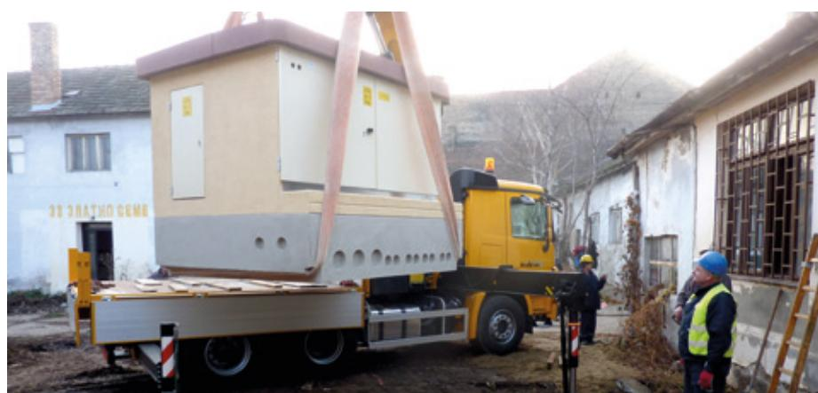
Istovar i ugradnja trafostanice / Discharge and installation of substation
