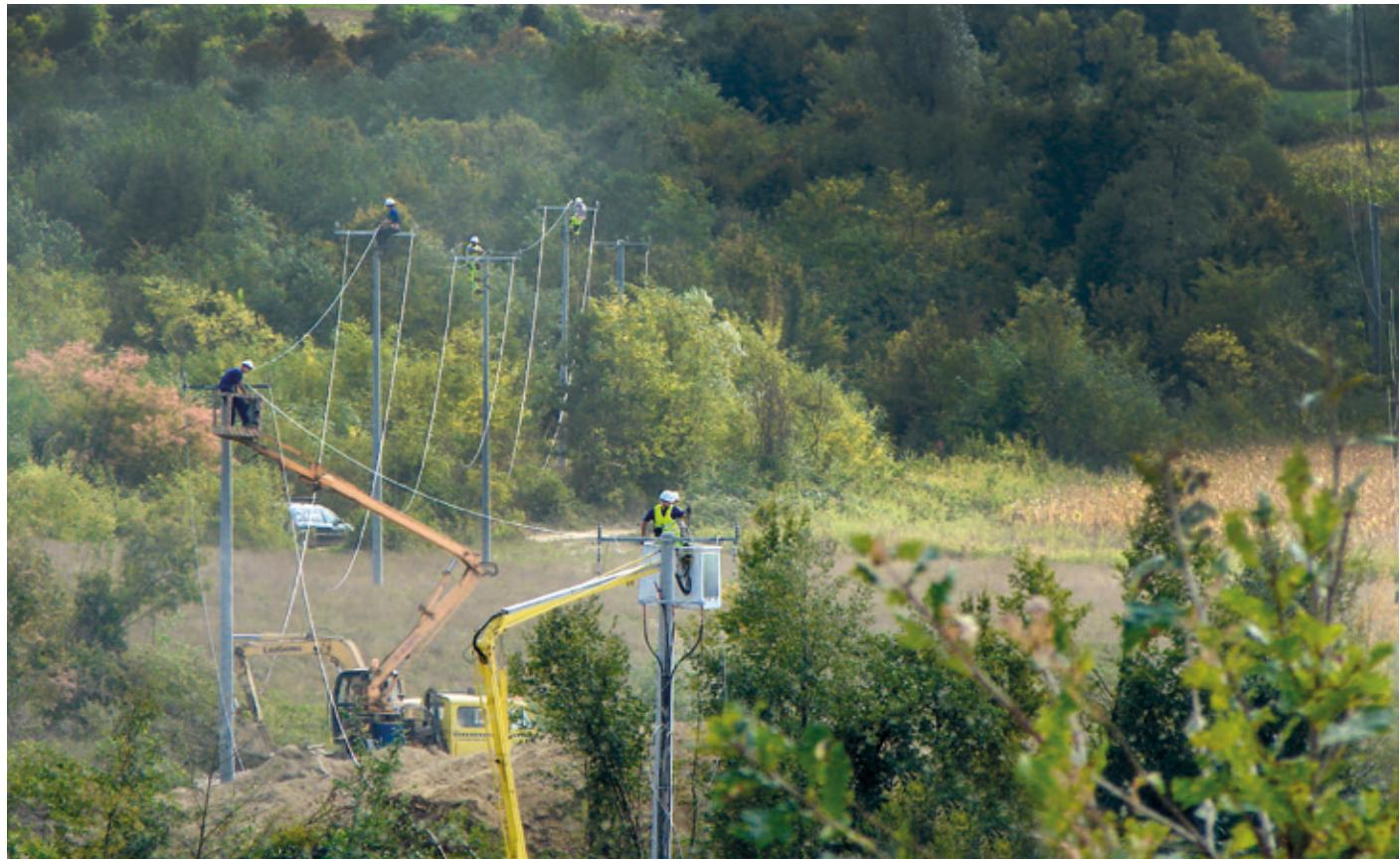
**Montaža ovjesne opreme i provodnika** / Installation of suspension equipment and conductors
