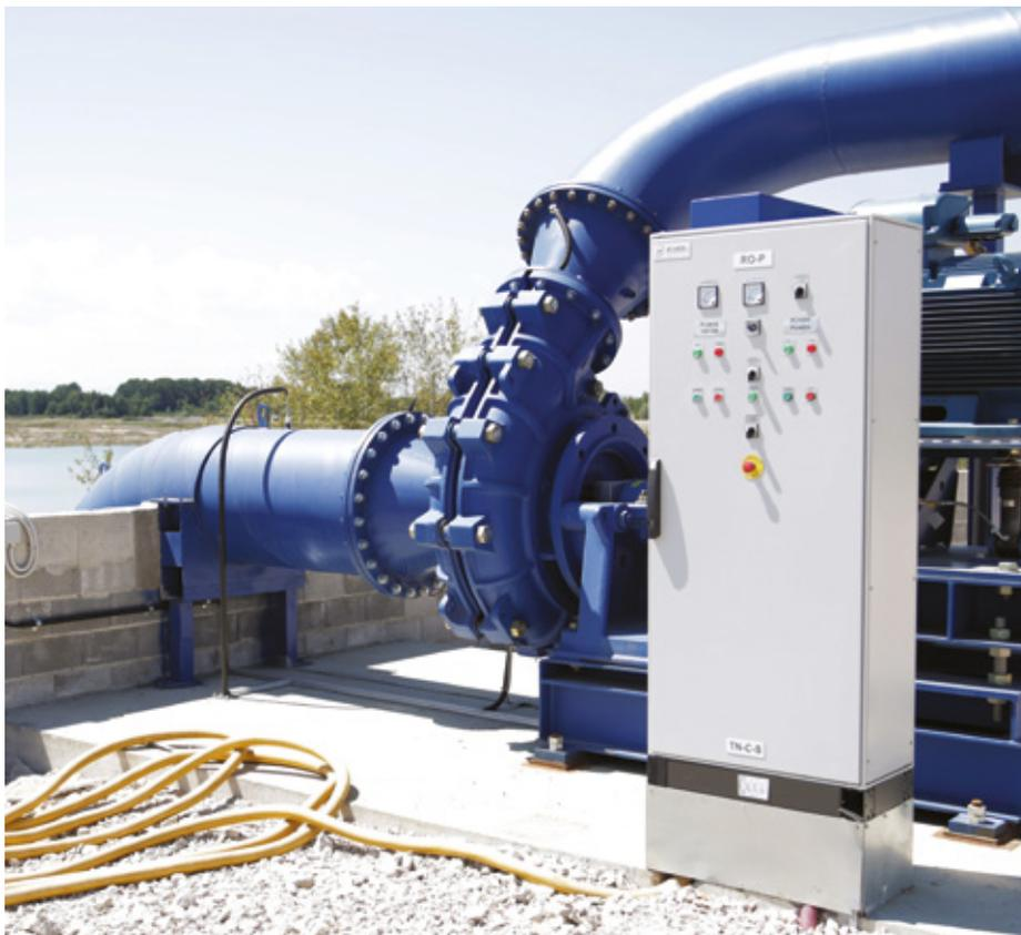
**Asinhroni motor 150 kW / Asynchrony engine 150 kW**
