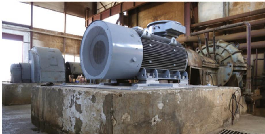
Asinhroni motor 500 kW / Asynchrony engine 500 kW
