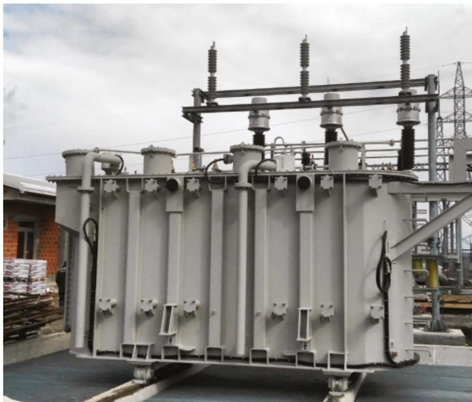
Novi energetski transformator snage 20 MVA / New energetic transformer, power 20 MVA
