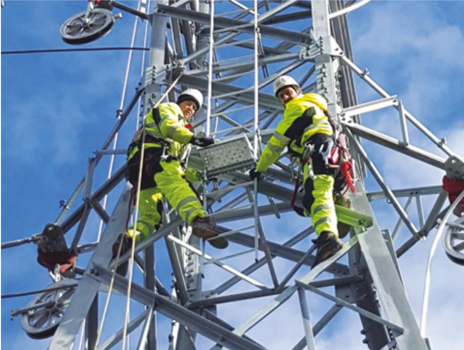
pletion of the project in planned deadlines. We performed transmission line entrance and exit to the substation, cut old transmission line, disassembled two poles, assembled and erected 11 new poles. Afterwards, we performed electrical assembly works and installed about 11 km of OPGW. Due to big number of crossovers, we performed works with robot's help, so called 'cable cat', and hence added another attractive work method in our rich biographies.
