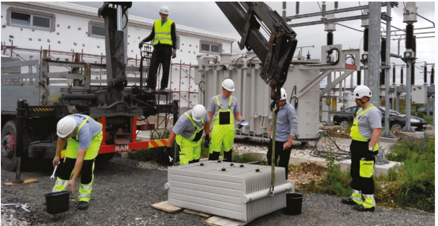
Montaža energetskeg transformatora / Assembly of energetic transformer
