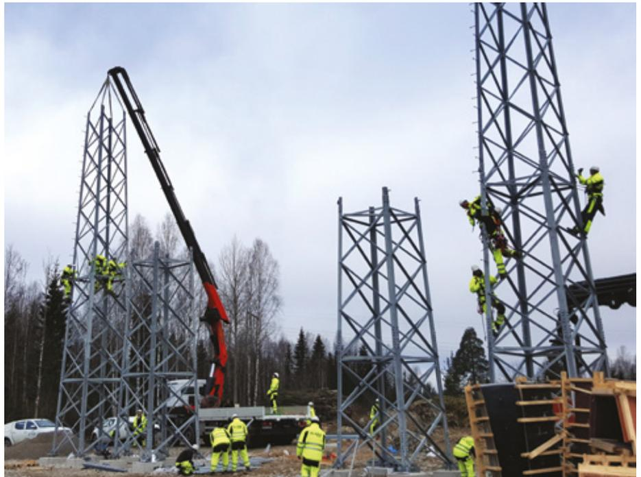
Podizanje stubova / Erection of poles
