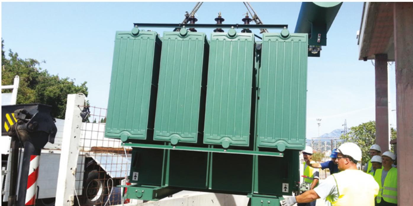
Istovar i ugradnja transformatora 35/10 kV, 8 MVA / Unloading and installations of transformer 35/10 kV, 8 MVA
