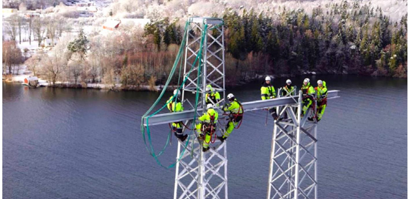
Montaža stubova 130 kV DV preko kanala Södertälje | Installation of 130 kV TL towers over the Canal Södertälje
