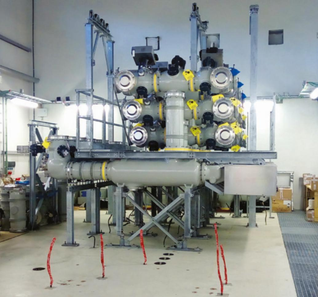
GIS 245/132/12 kV postrojenje u TS "Krafla 49" GIS 245/132/12 kV facility in SS "Krafla 49"
