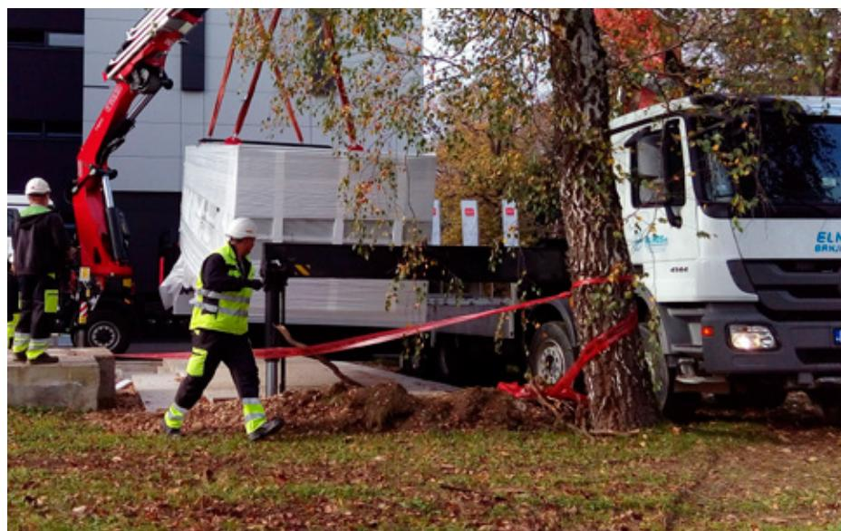
Agregat uspješno pozicioniran na temelj Generator successfully mounted on foundation
