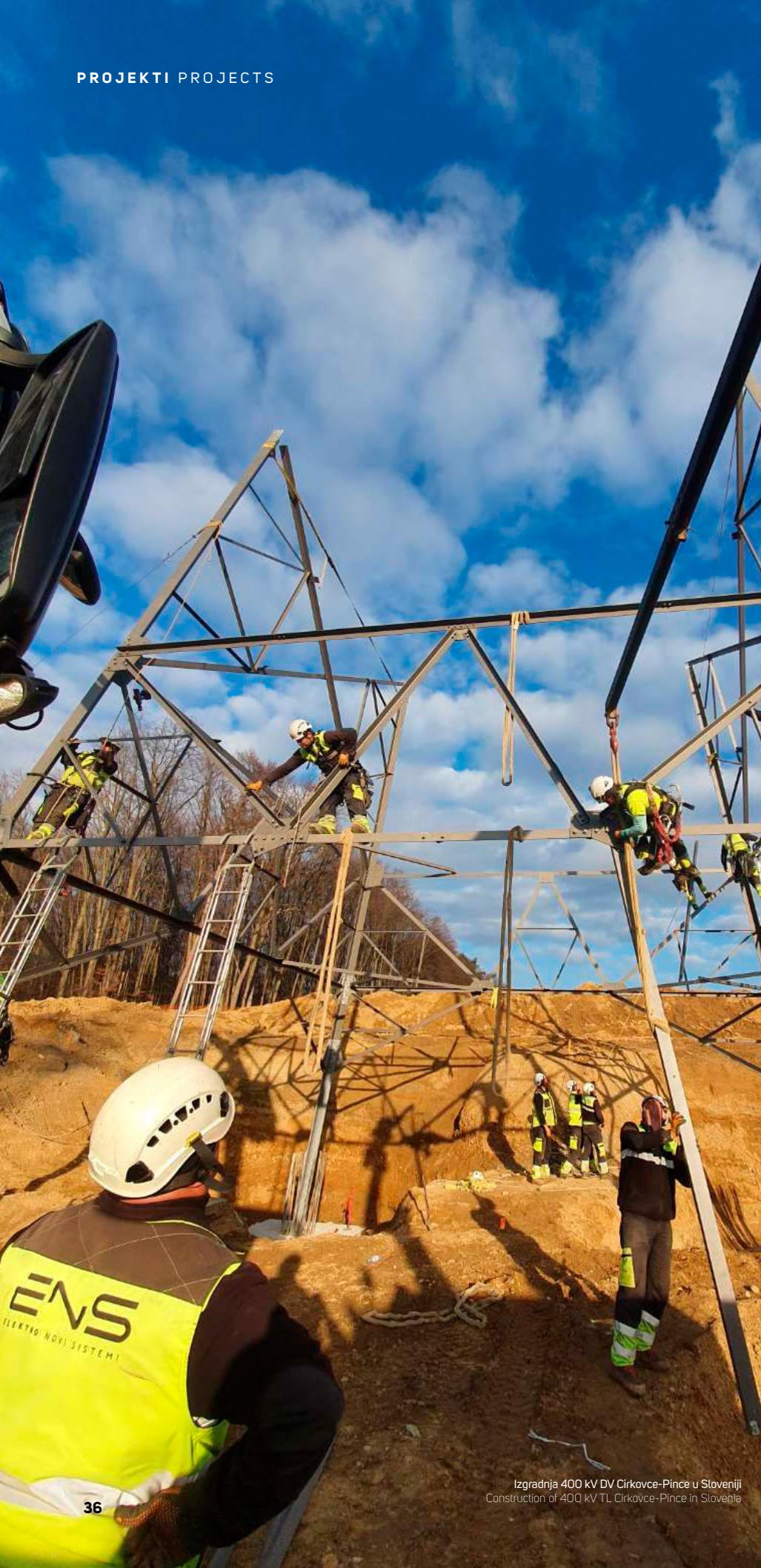
There were 138 towers set on the route of Hurva-Sege transmission line, and tower known under the name stubbe are the towers setting aside from the others by its size, weighing 55 tons and 55 meters high each. At the peak of the works performance, there were as many as 70 of our linemen working.
