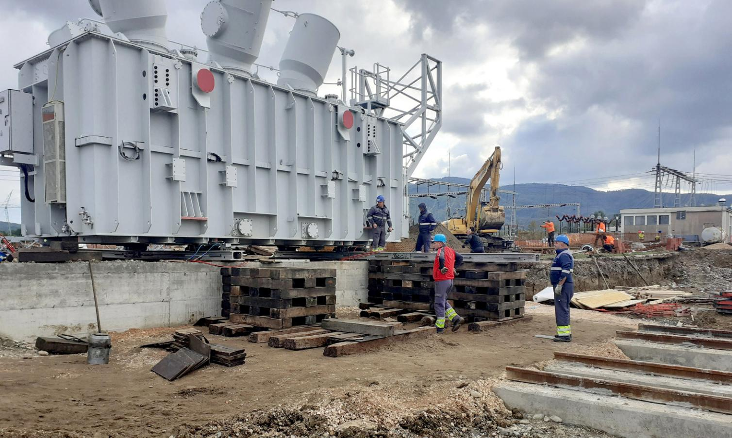
Transformator (400 MVA) teži 270 t Transformer (400 MVA) weighs 270 t
