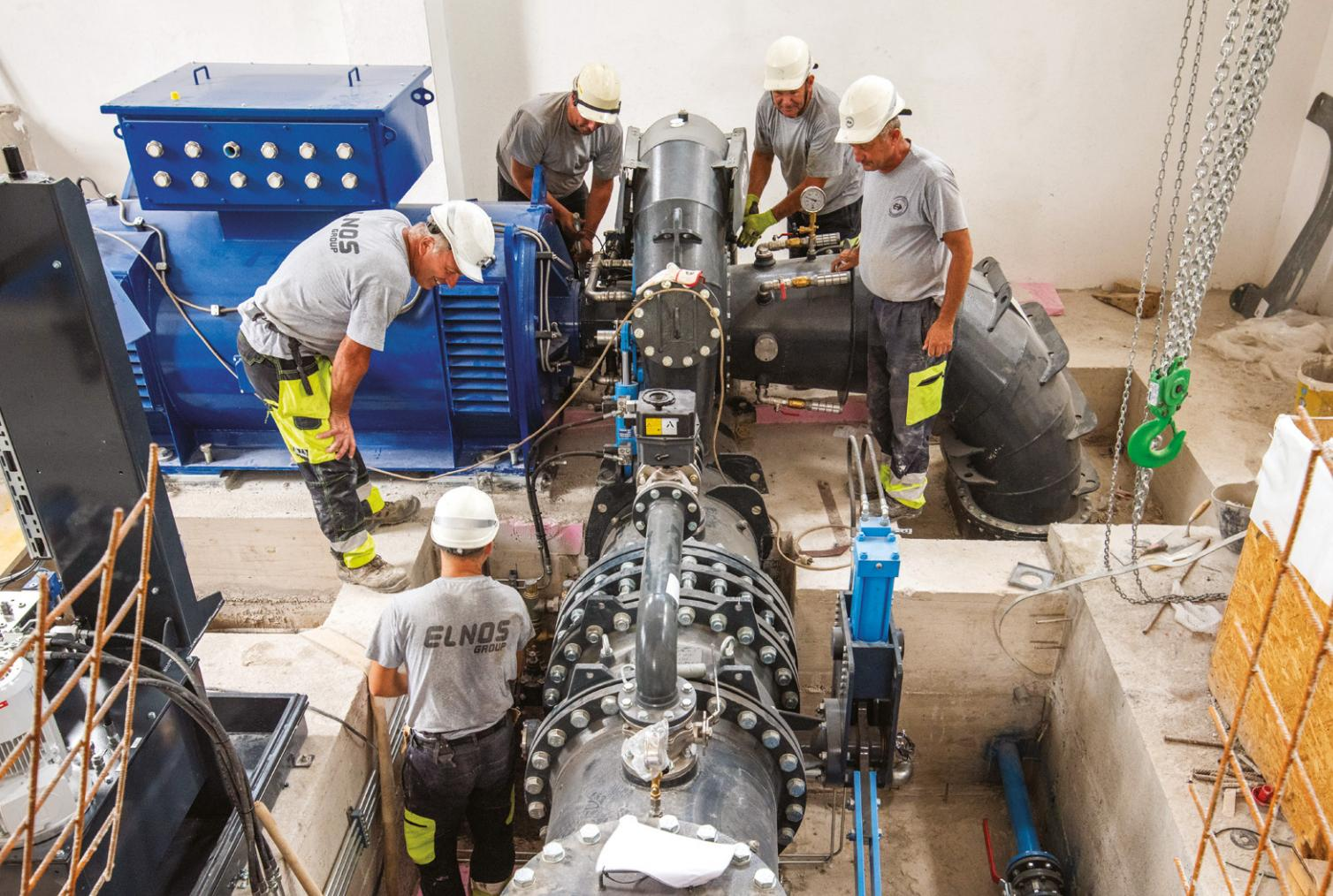
Ugradnja turbine i generatora u mašinskoj zgradi MHE Jablanica Installation of turbine and generator in mechanical building of SHPP Jablanica
