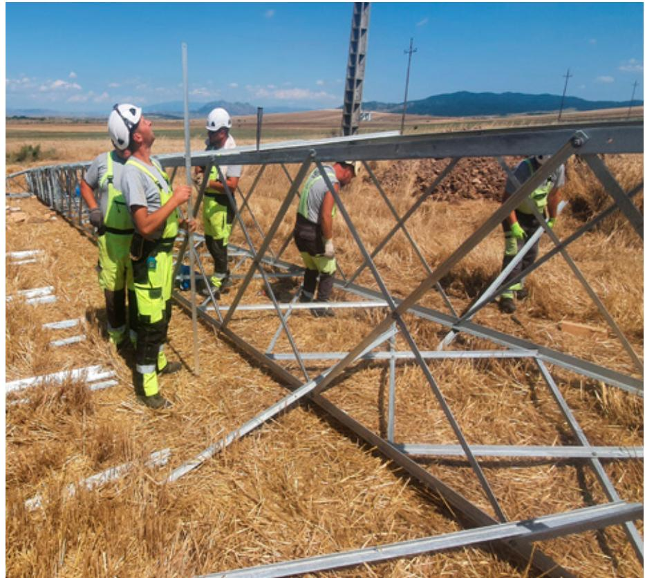
Throughout the summer, they dismantled the old and erected new-generation transmission line towers on extremely steep and challenging terrain. The new towers are designed and manufactured to withstand the harshest weather conditions.
