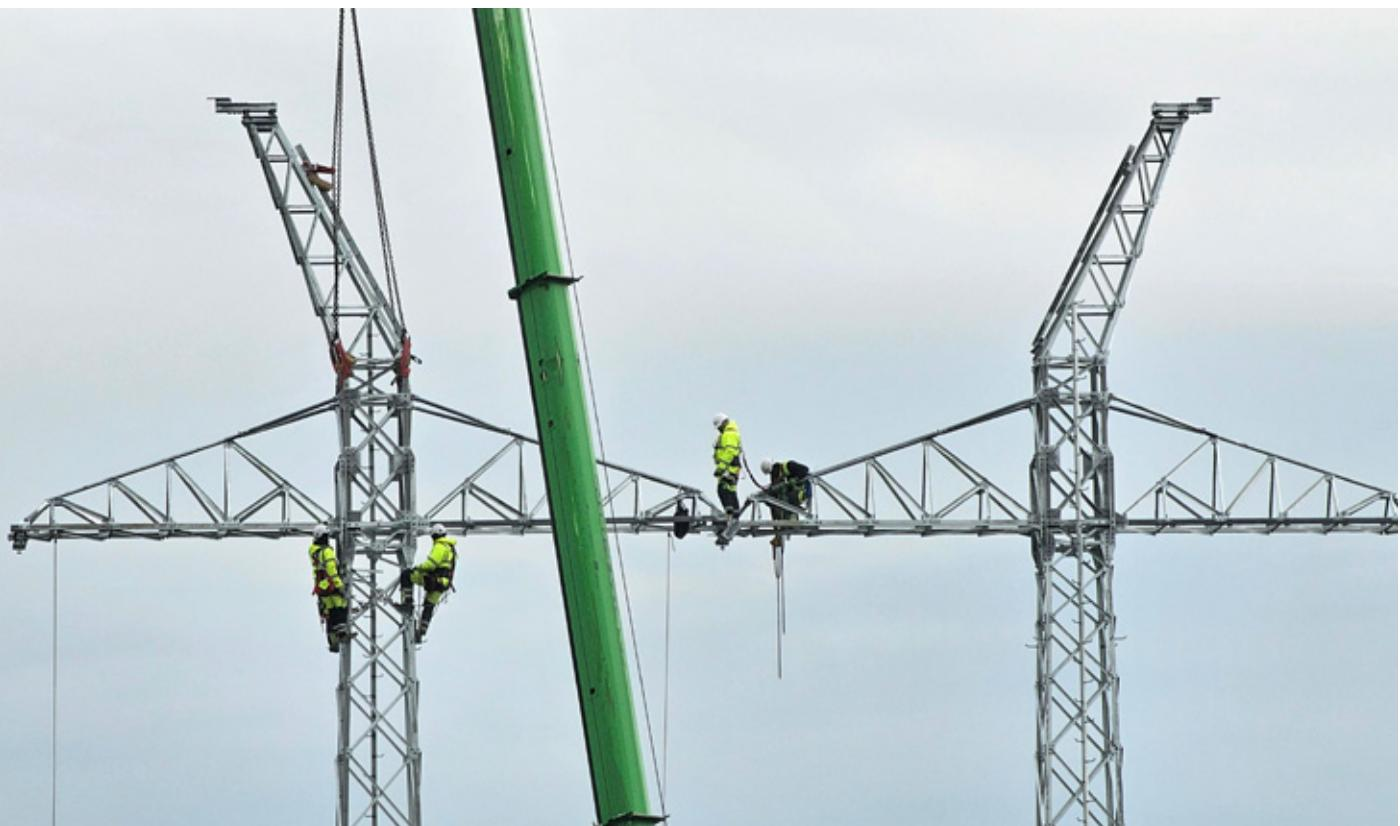
Rekonstrukcija 400 kV dalekovoda V-413 Reconstruction of 400 kV transmission line V-413
