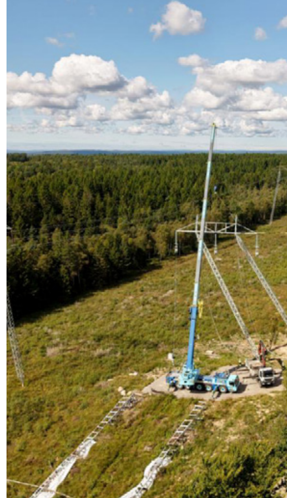
Radovi u toku Work in progress
