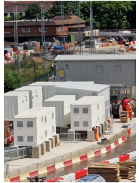
Gradilište projekta HS2 HS2 project site
